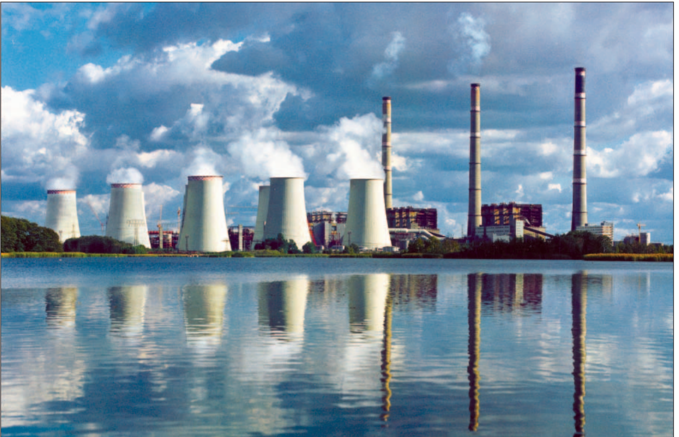
Reference example: VEAG Kraftwerk Jänschwalde with 6 turbo sets (500 MW each) and the ME 4012 turbine control system
