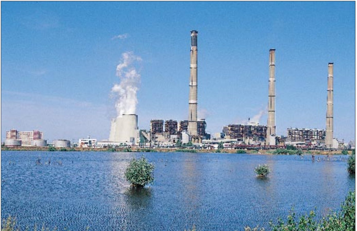
Kohlekraftwerk / Coal power station
