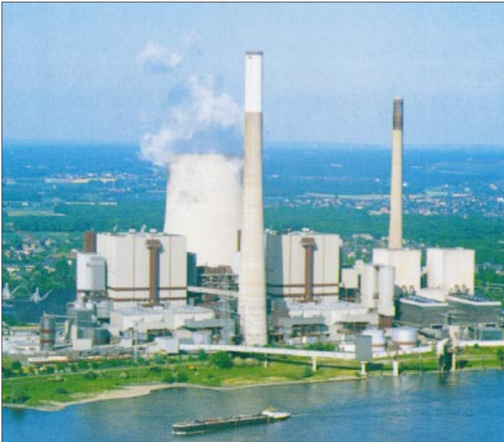
Kohlekraftwerk / Coal power station
