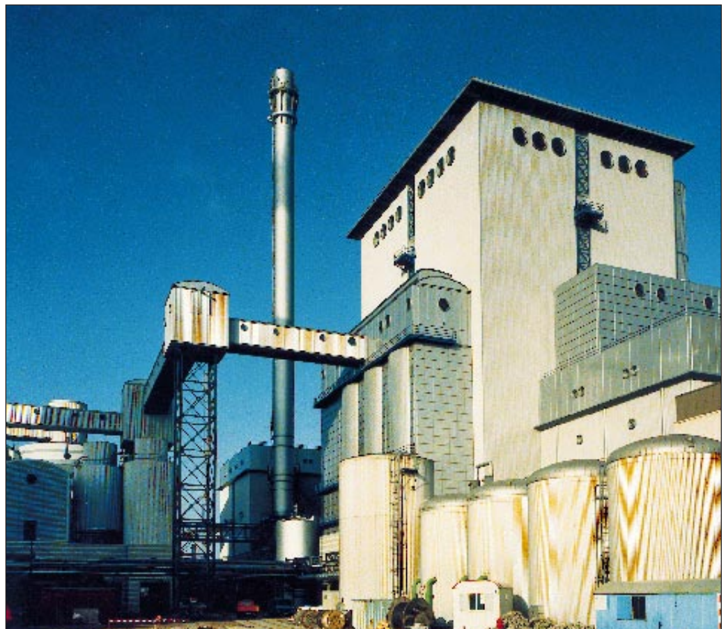
Heizkraftwerk / District heating power station
