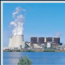
Power Station Control Systems
