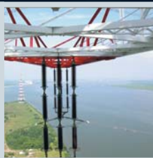
Power Distribution Control Systems
